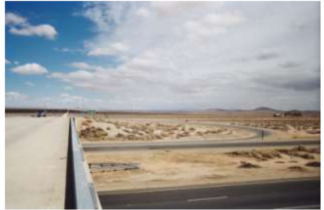
Photograph of Interchange Ramp (east of parcel) onto Westbound Highway 58
